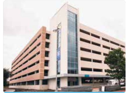
Methodist Richardson opened its new seven-story parking garage ahead of schedule in November.
